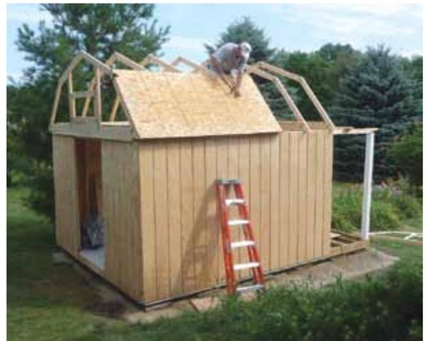
**Photo 1—Trusses designed to accept standard size sheets of roof sheathing reduce waste in both the truss itself and the roof deck.**
